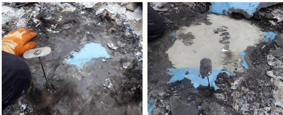
Figure 5: After the collapsed glass fleece and melted EPS insulation residues were removed, the undamaged vapour barrier (blue) on the cement-bonded particleboard was revealed.
