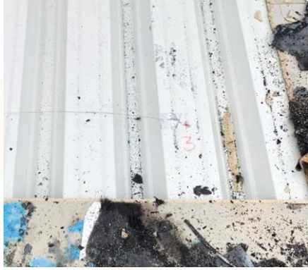
Figure 6: Below the undamaged cement-bonded chipboard, the trapezoidal sheet metal is also undamaged. The trapezoidal sheet has not been burned through.
