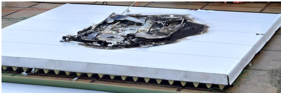
Figure 4: Flat roof with EPS foam and maximally overlapping glass fleece installation – The damage pattern demonstrates the effectiveness of the glass fleece and minimal fire spread underneath the completely destroyed PV system.
